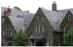
Fig. 11Ba. The tiles on the roof of this house are made from pieces of slate.
