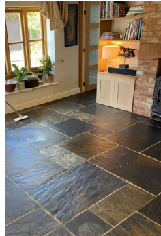
Fig. 11Bb. These floor tiles are made from slate tiles.
