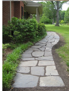
Fig. 11Bc. Slate tiles were used to create this walkway.
